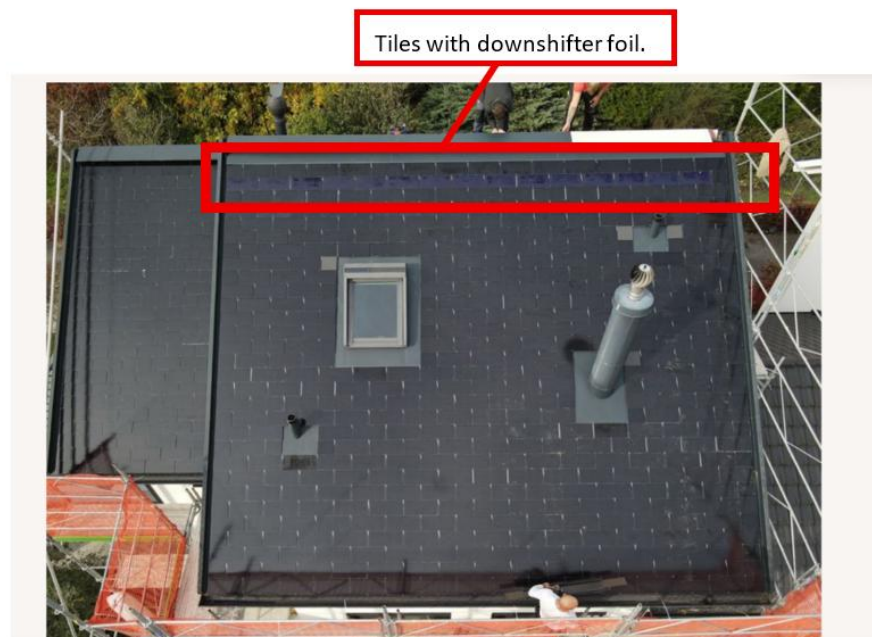
Figure 4 Downshifter tiles on the Founex demonstrator
